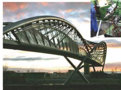
"Helix Bridge" Seattle, Washington 36" OD x 1.25" wall & 24" OD x 1" wall cold bent to a multiple radius helix
