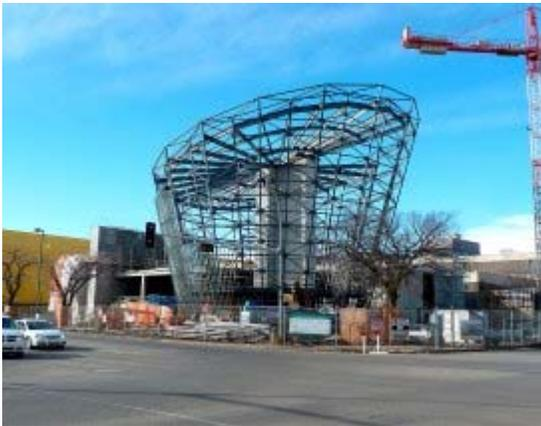
Cast Connex's Universal Pin Connectors were used in the assembly of the complex space frame of the University of Alberta's new Physical Activity and Wellness Centre. - Photo: ROBERT BOURDAGES, STANTEC
